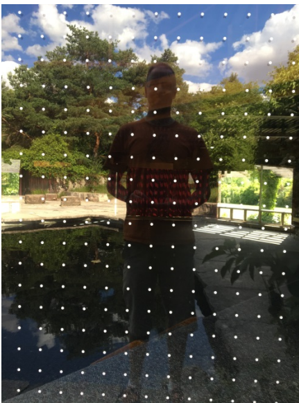
Take a look at how reflective windows can be! Birds just see the sky and trees because they have no understanding of what glass is and how reflections work. Adding dots will help them understand that it is a solid object Photo by Chris Earley
