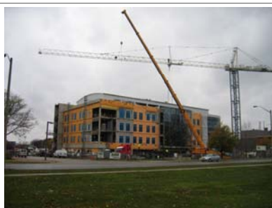
Removing the tower crane Oct 31- getting closer to the move Aug/2010!
