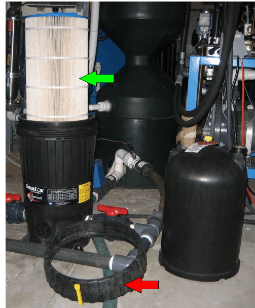
Open Filter: Red arrow indicates locking ring N.B. yellow tab. Green arrow indicates filter element
