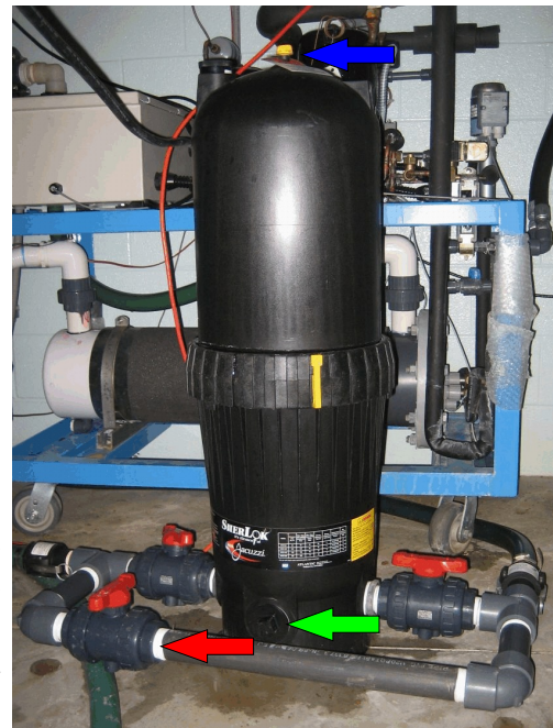
Jacuzzi SherLok Filter: Red arrow indicates bypass valve. Blue arrow indicates location of pressure relief valve. Green arrow indicates location of the drain plug
