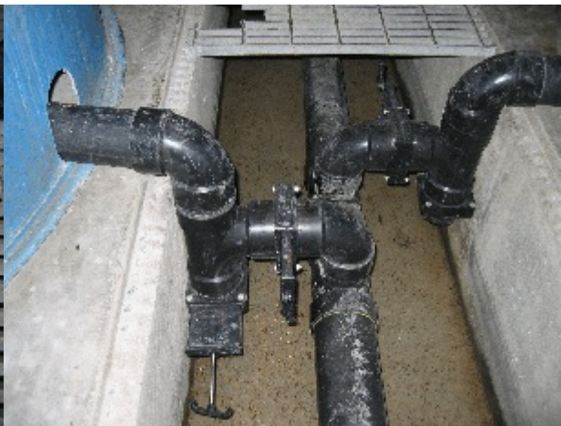
DRAINAGE TRENCH (grate removed)
