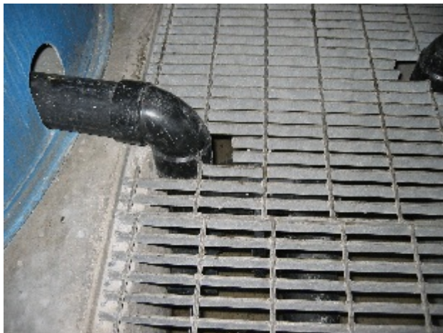
DRAINAGE TRENCH (with grate)
