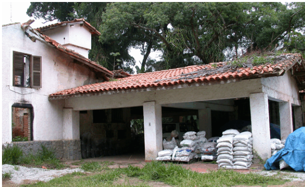
Figure 12. Carriage ports with walk through to backyard and rear of house.
