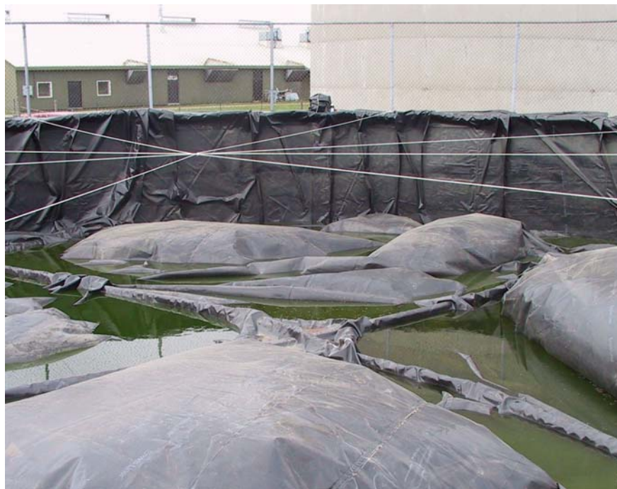
Figure 1. Pockets of gas under the NAP cover are removed by ducts connected to an exhaust fan. Water on top of the cover can be removed with a small pump. An agitation system using compressed air is installed on the floor of the storage.
