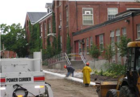
New wheelchair ramp for CPS off a new Trent Lane, August 2009.
